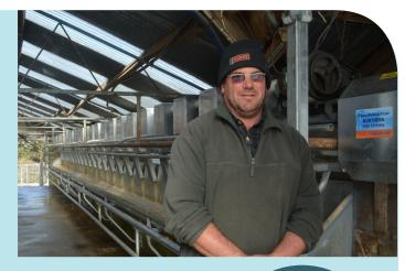
The new feed silo and hopper for lead feed, complete with automatic cut offs, have streamlined the feeding process. "Without the hopper, I'd have to walk out to the silo with buckets and fill them up. This has made the dairy easier to use."
